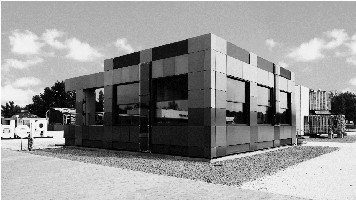
Figure 10. MOR building. The facility is located at The Green Village in the TU Delft campus. This building was utilised for experimenting.
